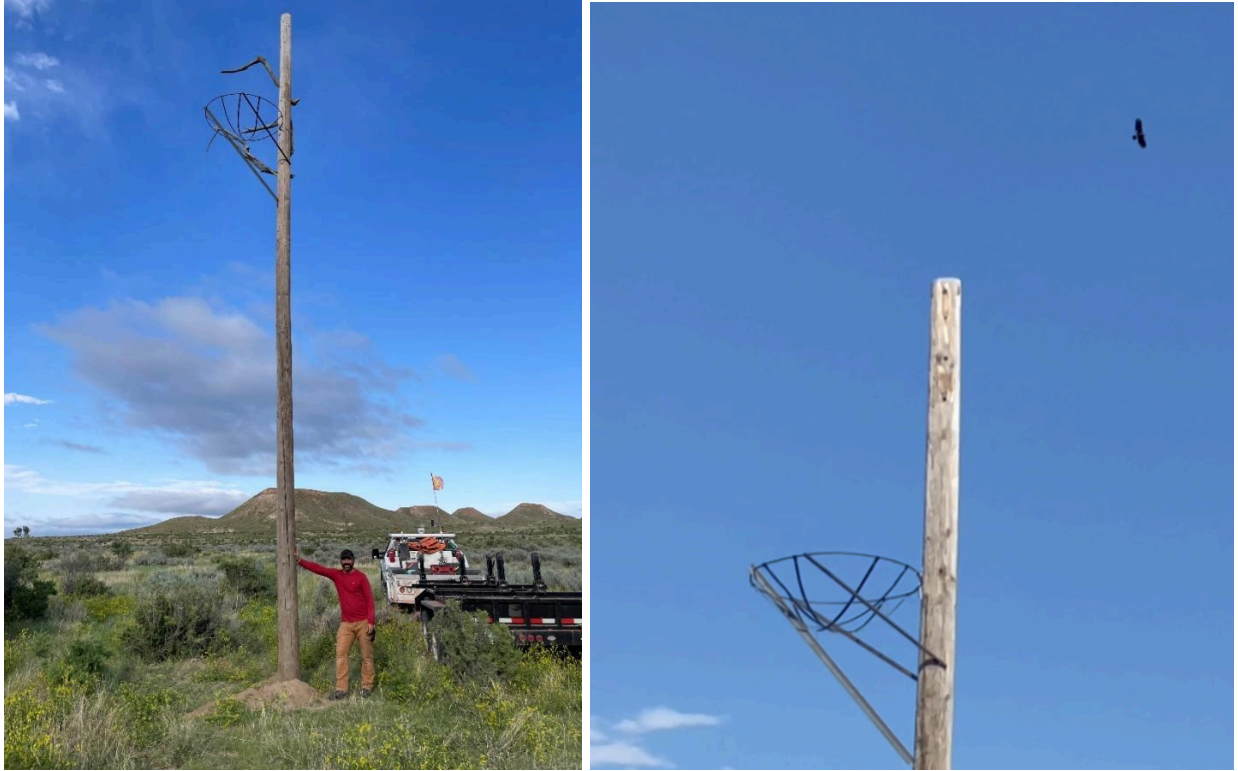
Figure 4. Examples of initial pole installation for artificial nesting structures placed in the Great Plains for golden eagles (left). Golden eagle flying over pole during installation process (right).
