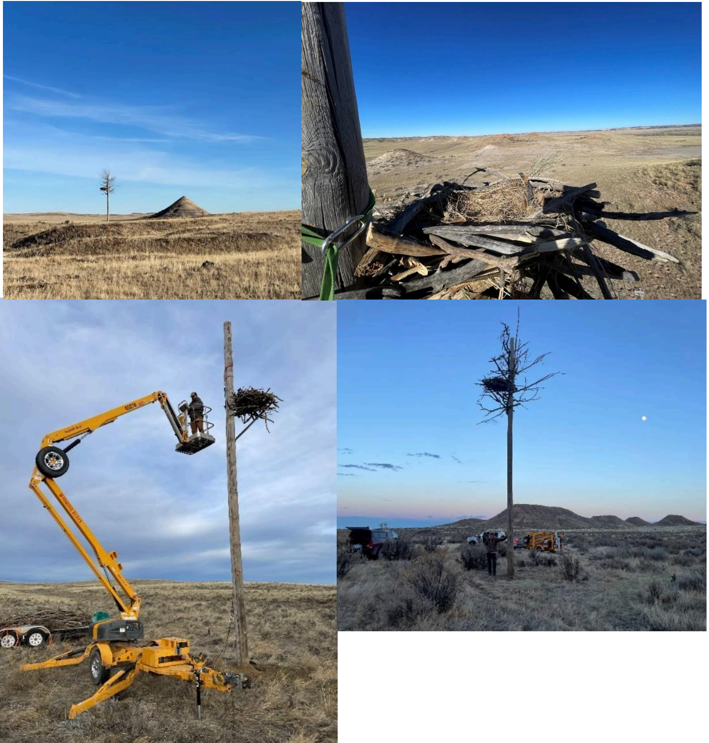
Figure 6. Examples of artificial nest structures (and their final installations) using retired utility poles.
